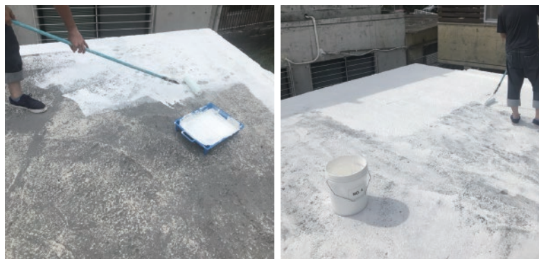
Pictures during painting work
